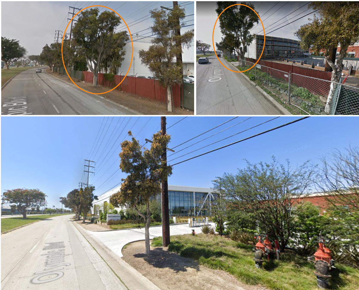
Restitution resolved, posted and removed for Fire & vehicular access at the "Pen Factory" remodel 2701 Olympic Blvd.
