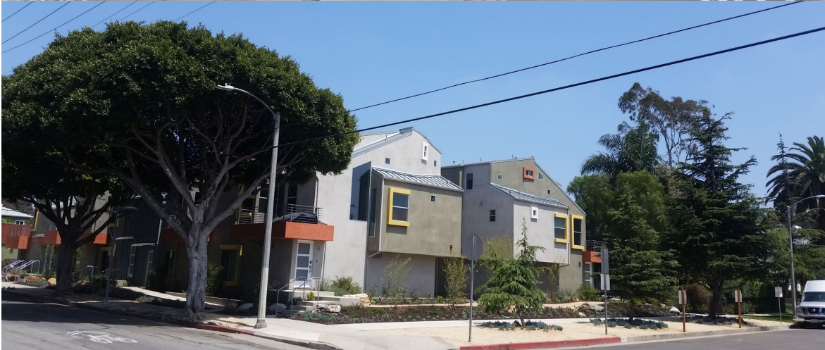
South-East Corner of Michigan Ave & 16 th st
