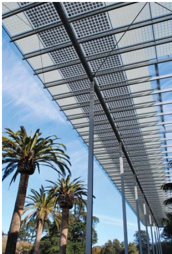
SOLAR PANELS PROVIDE SHADE OVER WALKWAYS AND PARKING
