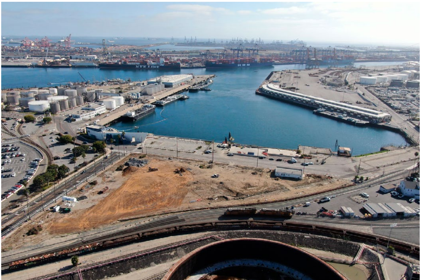
Construction begins on Wilmington Waterfront Promenade
