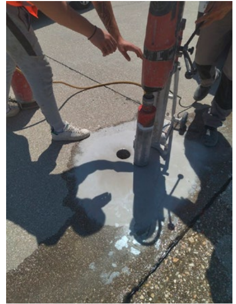
CONCRETE CORING ON SITE
