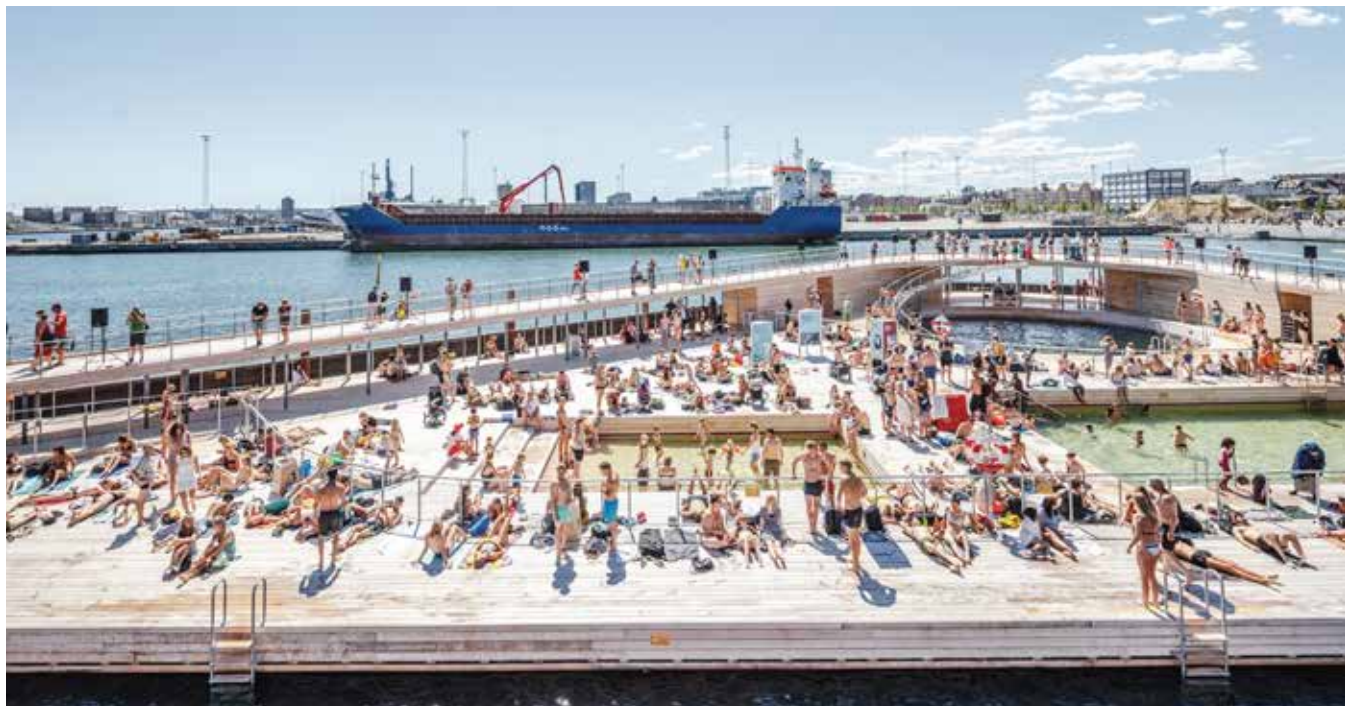
AARHUS HARBOR BATHS EXTENDS PUBLIC SPACE INTO THE WATERS OF THE CITY.
