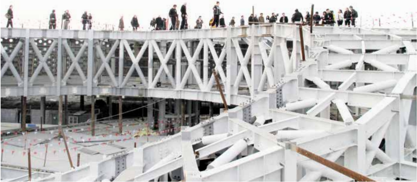
DANISH PAVILION FOR THE 2010 WORLD EXPO IN CONSTRUCTION
