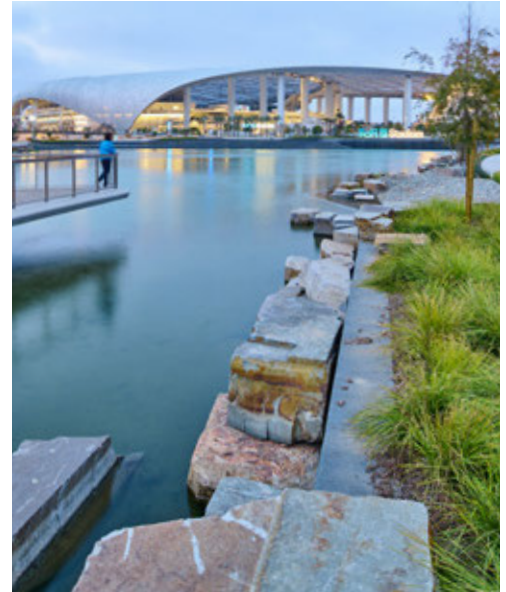
Hollywood Park Redevelopment, SoFi Stadium — Inglewood, CA
