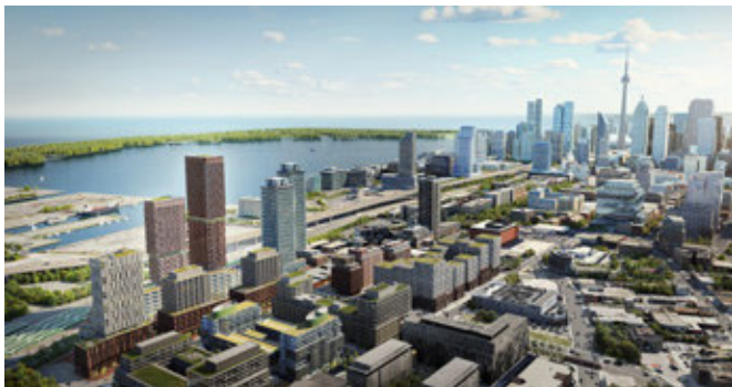
Block 20 Mixed-use Development — Toronto, ON, Canada Project Role: Project Manager
