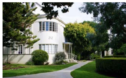
San Vicente Courtyard Apartments, Historic Context Statement and Evaluation Santa Monica, CA
