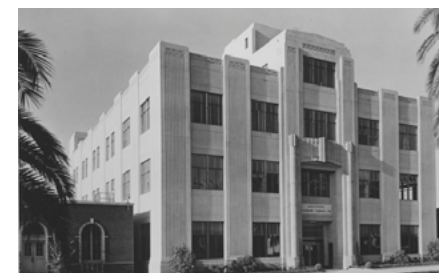
Associated Telephone Company Building, Landmark Nomination and Mills Act Contract Santa Monica, CA
