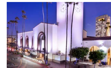
Los Angeles Union Station, Historic Structures Report and on-going Historic Preservation Consultation Los Angeles, CA
