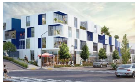
2903 Lincoln Boulevard—New Mixed Use Project Santa Monica, CA
