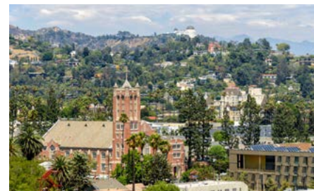
City of Beverly Hills – Climate Action and Adaptation Plan Beverly Hills, CA
