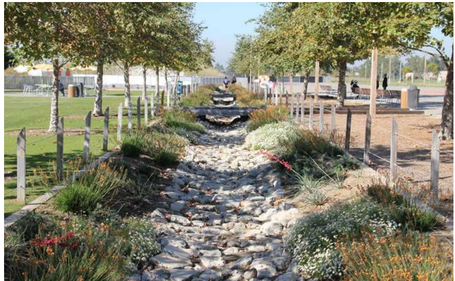
THE PARK USES NATURAL WATER TREATMENT SYSTEMS TO CLEAN URBAN RUNOFF AND REUSE IT FOR IRRIGATION TO REDUCE DEPENDENCE ON POTABLE WATER. 3.5 MILLION TONS OF CONCRETE AND STEEL WERE SALVAGED & RECYCLED FOR CONSTRUCTION MATERIALS.
