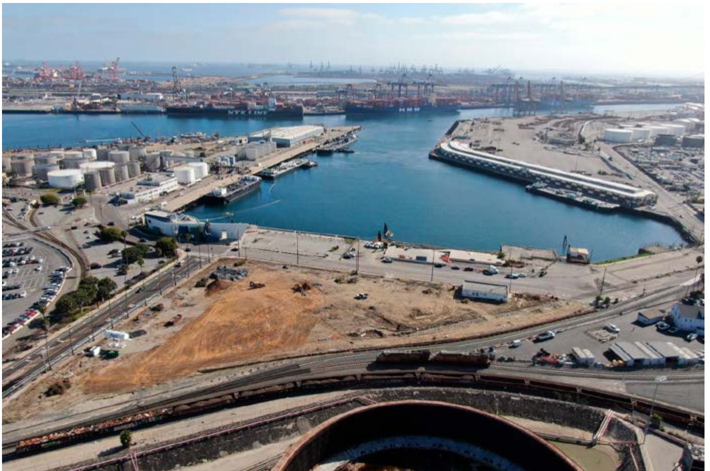
Construction begins on Wilmington Waterfront Promenade
