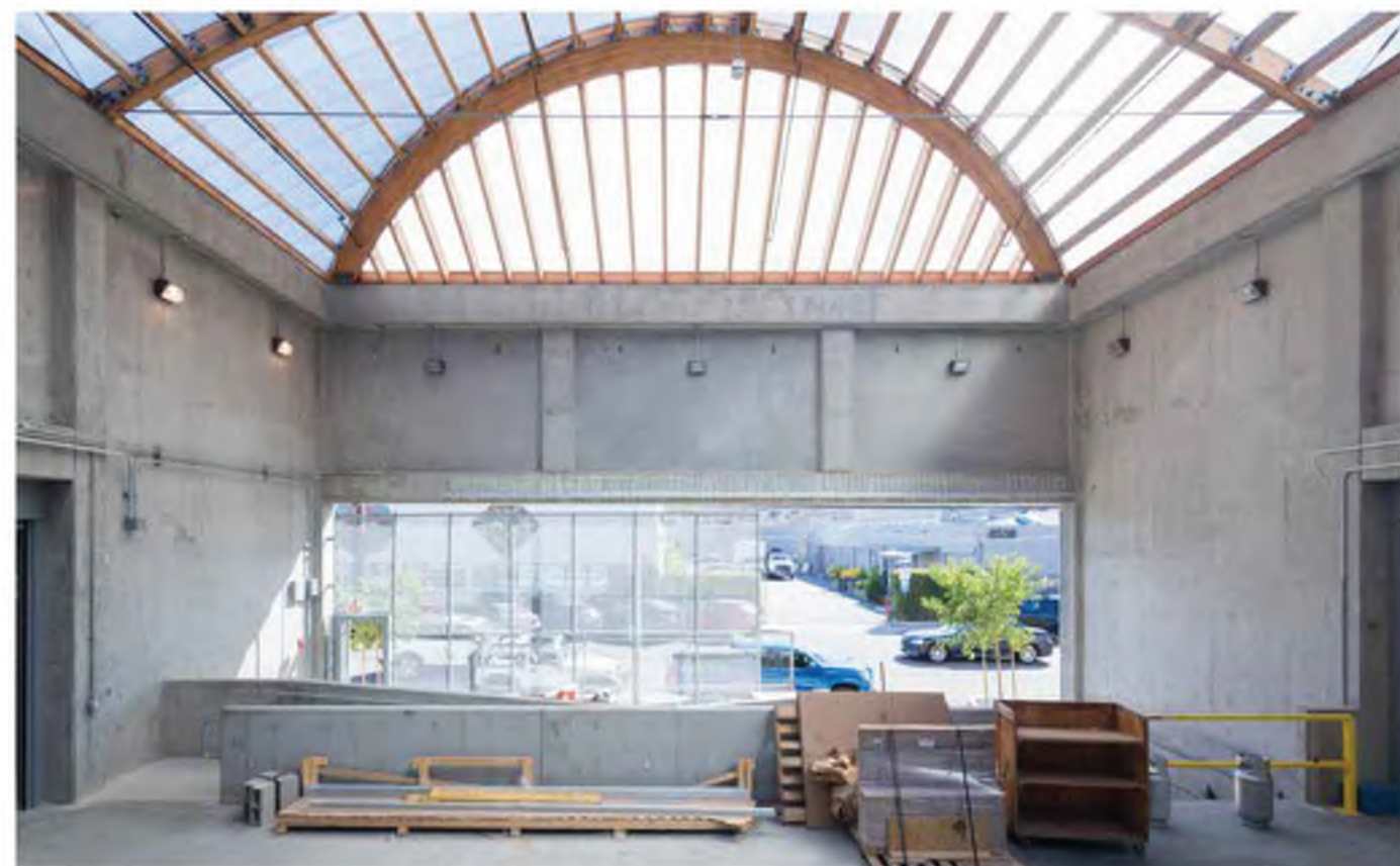
Exterior sculpture yard (above), Loading and ceramics yard to street beyond (below)
