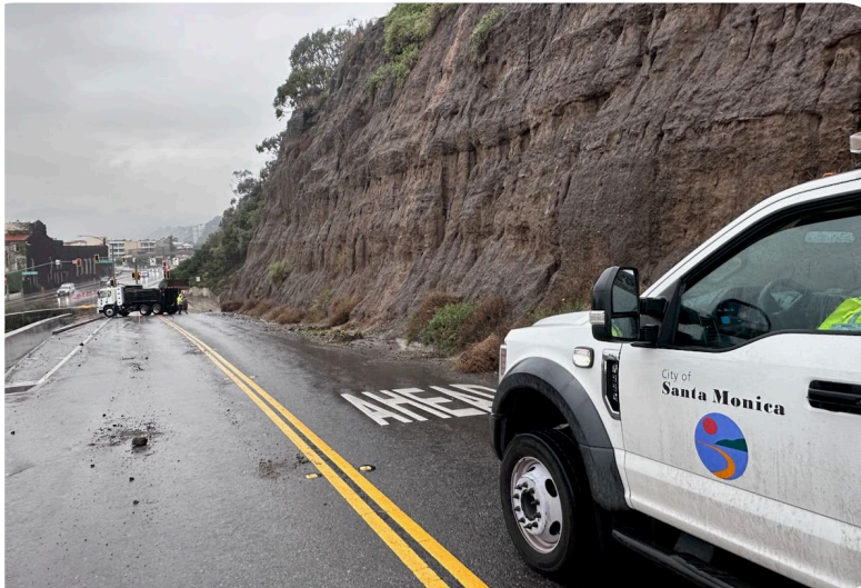
Slope stability work on the Palisades Bluffs in February 2024
