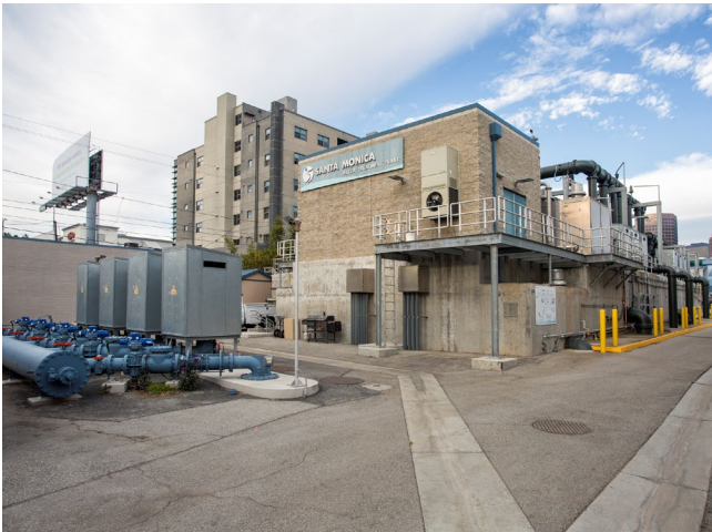
Historically, Santa Monica's groundwater supply has been negatively impacted by leaking underground storage tanks which caused contamination of the Charnock and Olympic groundwater wells during the late 1990s to early 2000s. The contamination is being addressed using filtration with granular activated carbon to treat water from three contaminated wells, followed by additional treatment at the Reverse Osmosis (RO) facilities at the Santa Monica Water Treatment Plant.
