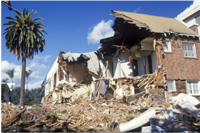
Damage from the 1994 Northridge earthquake
