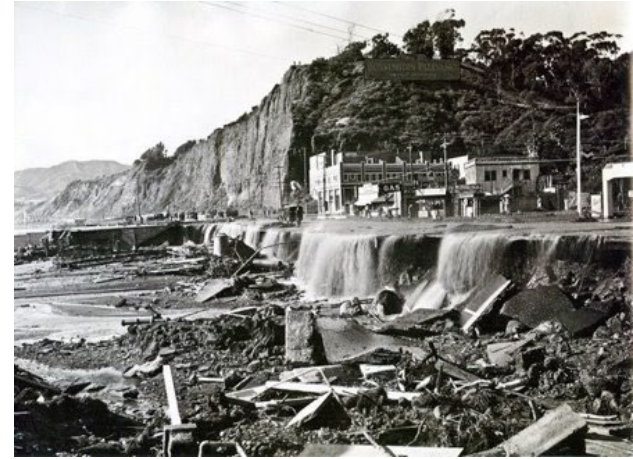
Damage from the 1938 flood at Santa Monica Canyon
