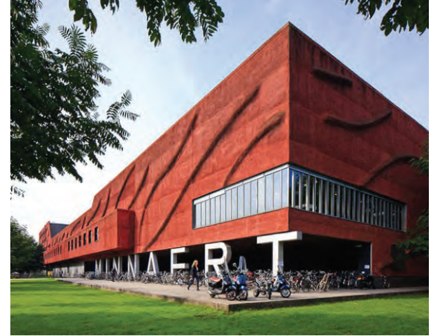
Playful and engaging signage is effectively integrated into the architecture of this contemporary building
