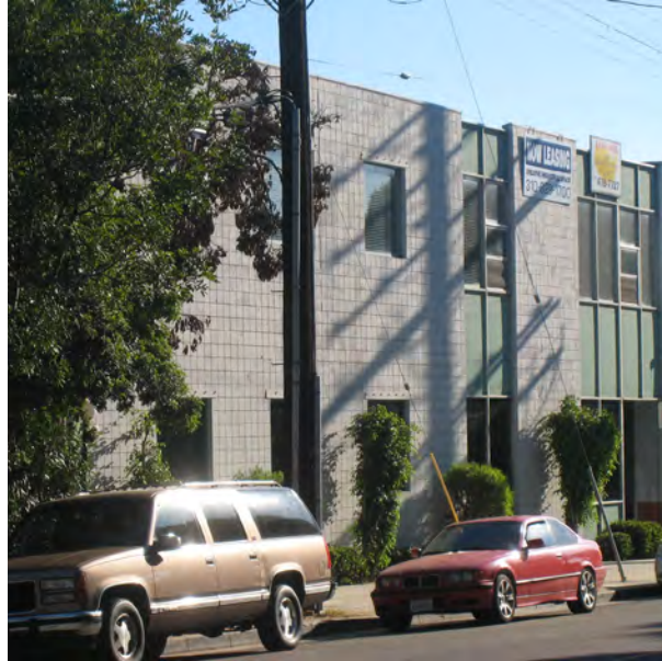
Local Connector Street: Nebraska Avenue near Stewart Street.
