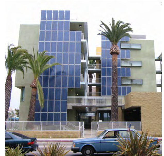
A wide range of housing options will allow more area workers to both live and work in Santa Monica, reducing commute times and total vehicle miles traveled.
