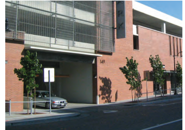
A parking garage in Petaluma with a single lane entrance leading to multiple access lanes within the garage that help to minimize the width of the streetfront garage entry.
