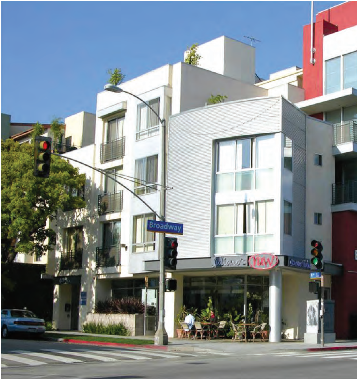
Ground floor entries and the balconies for the upper floor dwelling units are oriented along the public rights-of-way to support the pedestrian realm in this Downtown Santa Monica building.
