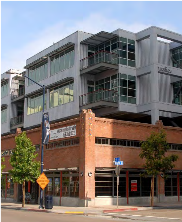
An industrial structure in San Diego, CA has been expanded with new uses while the historic brick facade has been preserved to maintain its character.
