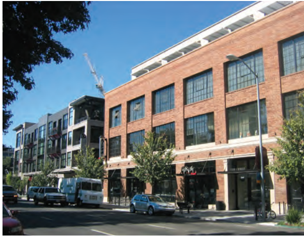
The structural bays of this mixed-use building provide scale and rhythm along the street.
