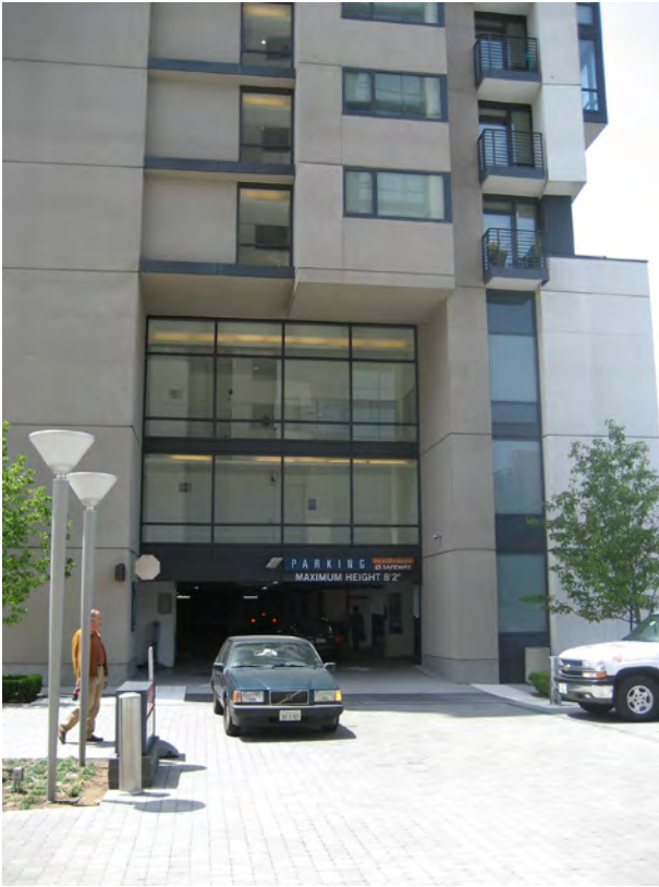
Private parking garages will include mostly shared parking spaces to support the Plan area's "Park Once" strategy.
