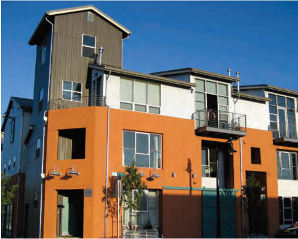
Upper floors of this apartment building are designed to increase solar access and air circulation within the units.
