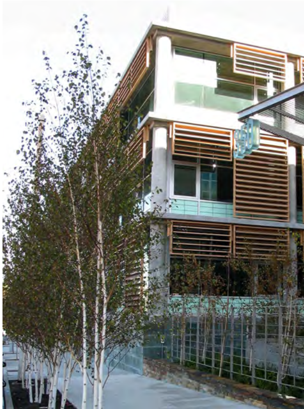
Innovative architecture with sustainable building design and creative materials is encouraged for the Bergamot Plan area.
