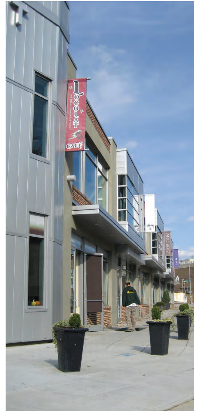
A corrugated metal facade on this building relates to industrial contexts.
