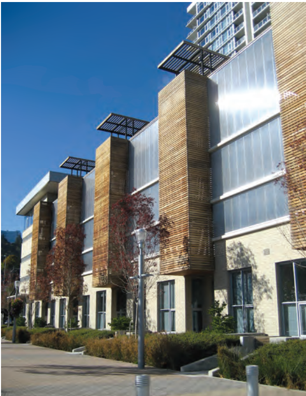
Modulated facade and ground floor uses activate this parking structure.
