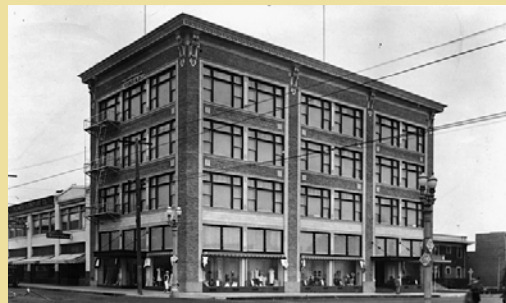
The Henshey’s building, built in 1924, was critically damaged in the earthquake. This site is now the location of R.E.I.
