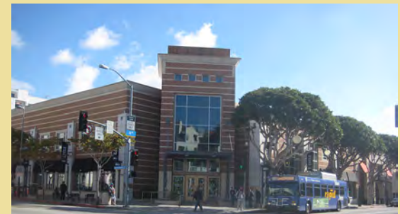
R.E.I. (formally Toys”R”Us) replaced the earthquake-damaged Henshey’s building.
