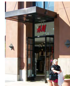
Canopy materials are durable, complement entry materials/colors and provide opportunity for recessed lighting at entry.
