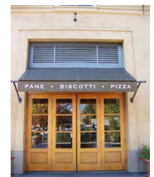
Shuttered wood awning adds texture to building façade and provides durable surface to add signing.
