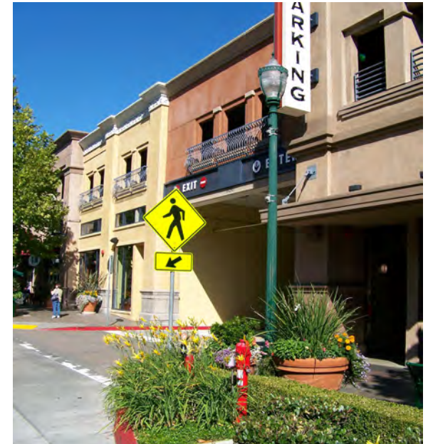
French balconies add architectural interest to upper floors of garage.
