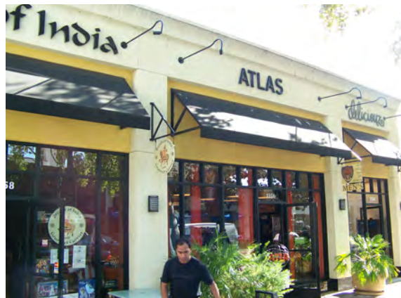
Awning color-coordinated with brackets, signs and light fixtures add harmony to the façade, but is too shallow to provide meaningful shade for shoppers.
