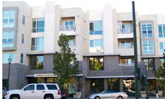
Color variation differentiates the building base from body. Offsets and recesses along the façade break up the building’s mass.
