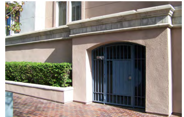
Decorative enclosure built into building façade can screen transformers and other utilities in an attractive manner.
