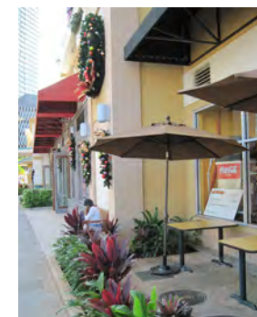
Awning design is consistent along business windows to reinforce identity of space.
