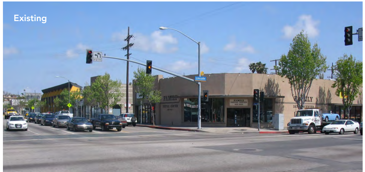
The intersection of Lincoln Boulevard and Pico Boulevard is where proximity to I-10 results in some of the highest traffic volumes in the City. Current development is auto-oriented and lacks architectural identity.
