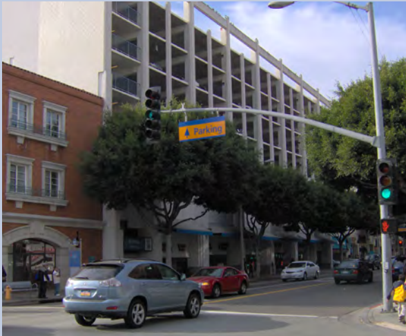
Evaluating performance measures—such as intersection capacity—will help determine how well the transportation system is operating.
