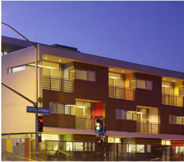
Affordable and workforce housing is highly desirable.
