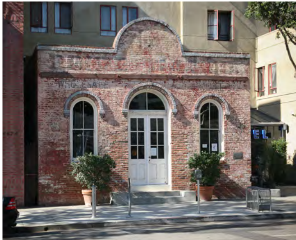
Adaptive reuse of historic buildings acknowledges that change can occur while preserving Downtown's history.
