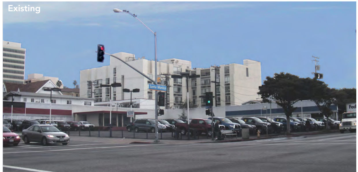
The existing automobile dealership format includes surface parking on the street frontage that does not actively engage the public.
