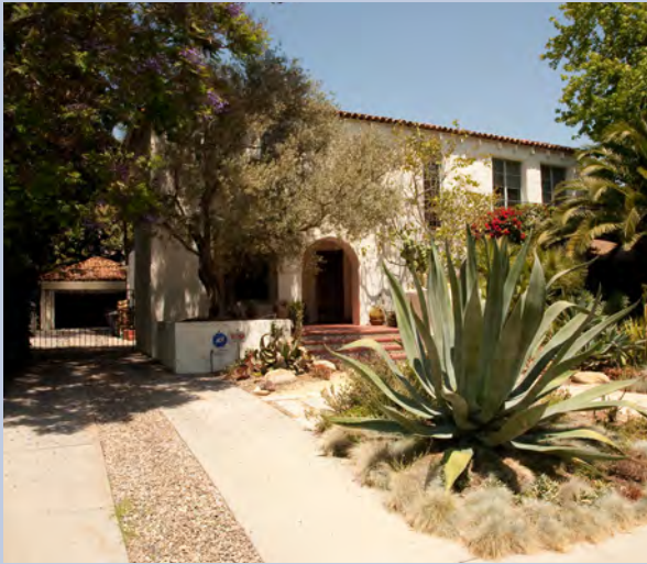
The Gillette Regent Square area contains a concentration of important residential structures that speak to Santa Monica's rich past.
