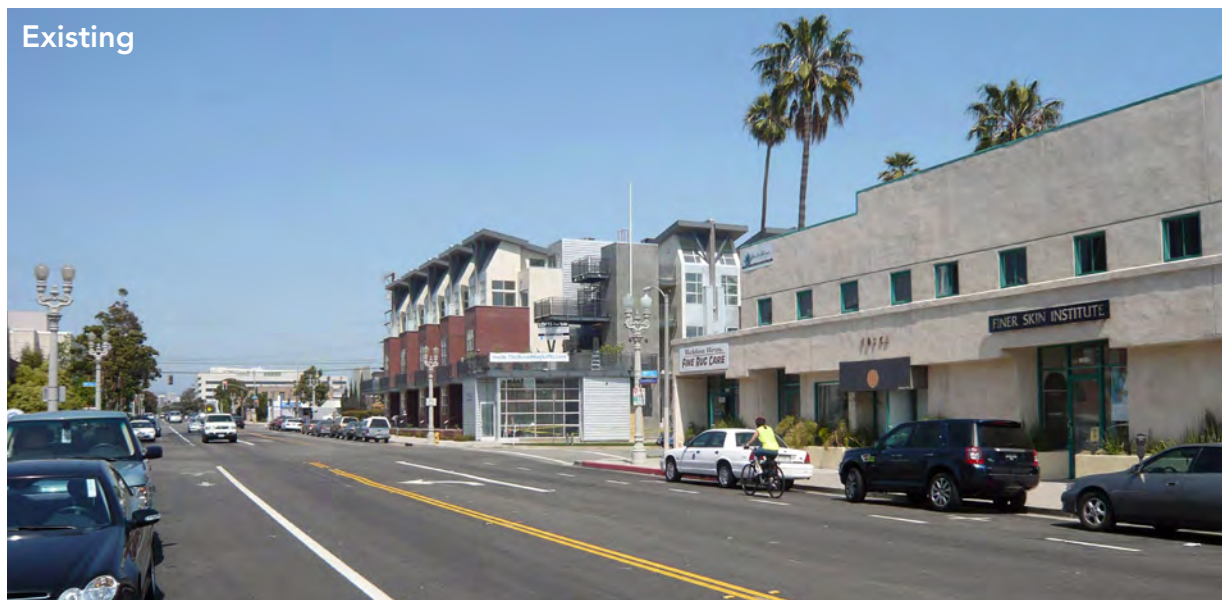
Broadway’s built environment is aging, and does not engage the bicyclist or pedestrian consistently along the street.
