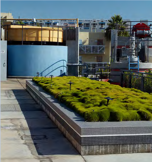
Water quality is a major resource issue, and one that Santa Monica takes very seriously. The SMURRF, pictured above, treats dry weather urban runoff before it enters the Bay.
