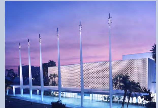
The Santa Monica Civic Auditorium has been host to many cultural events over the years. It has the potential to serve as a key component of the City's future cultural programming.
