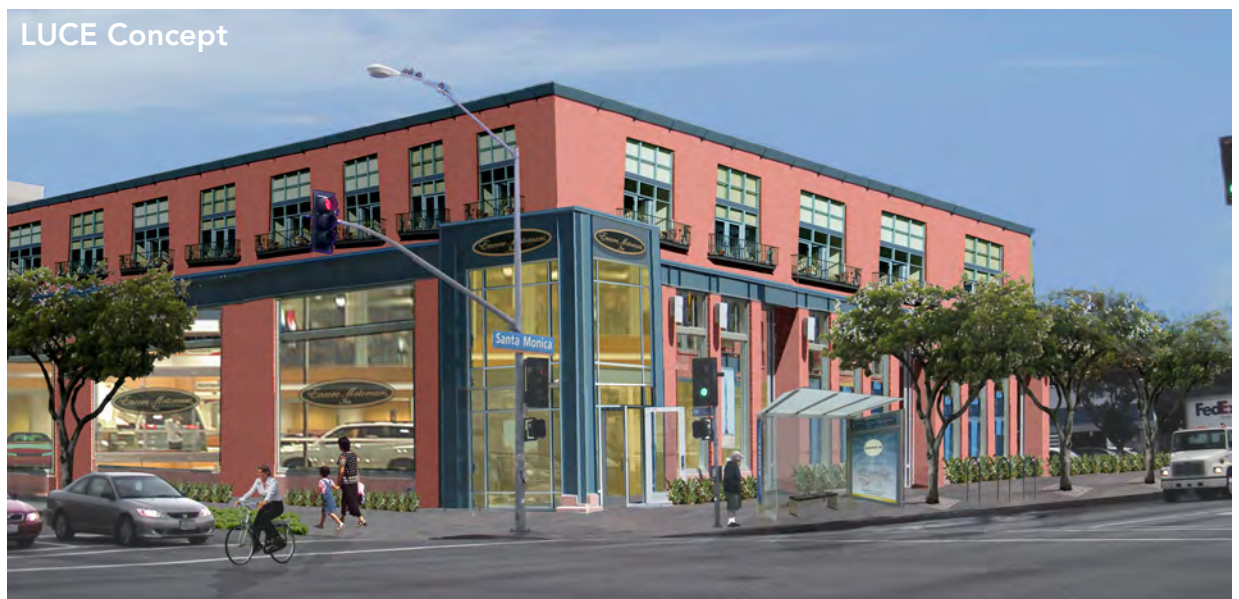
The LUCE recommends rethinking the showroom and service facility design of automobile dealerships.
