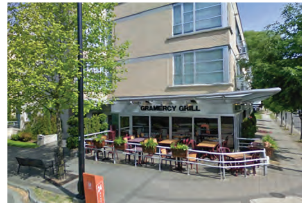
New requirements for TDM measures should be included in modifications to the Zoning Ordinance.
