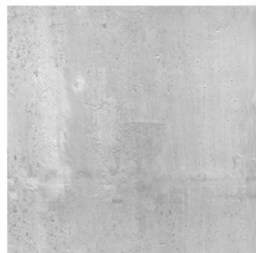
SMOOTH EXPOSED CONCRETE
