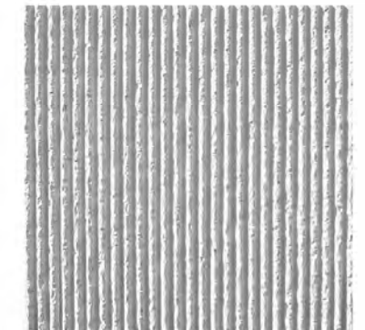
FORM LINED EXPOSED CONCRETE
