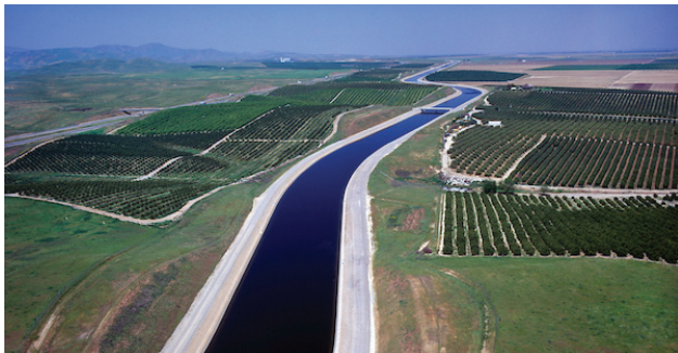
The California Aqueduct in the Central Valley.
