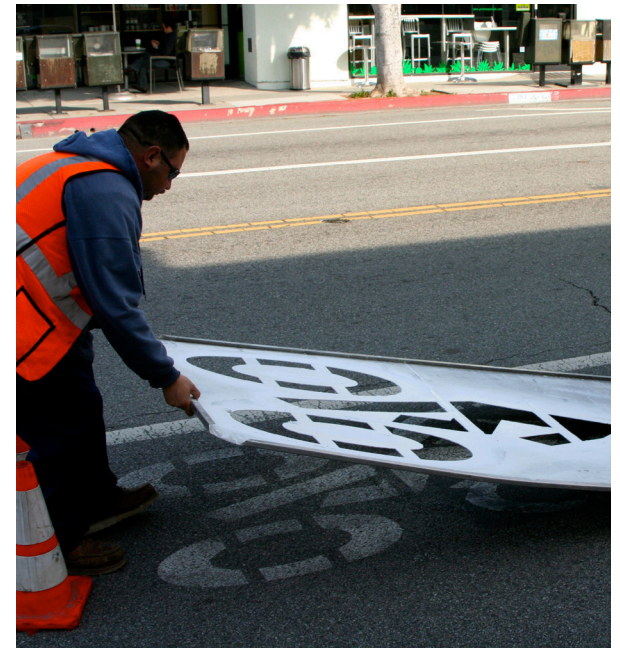
City crews install bicycle lane symbols and directional arrows.
