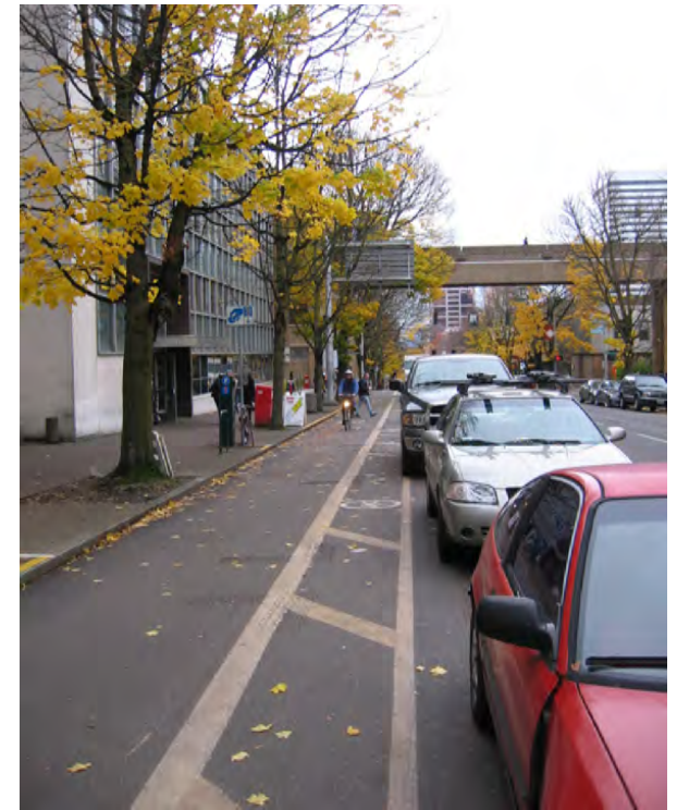
Cycle tracks offer cyclists protection from traffic with marked buffers and on-street parking. Source: Nelson\Nygaard
