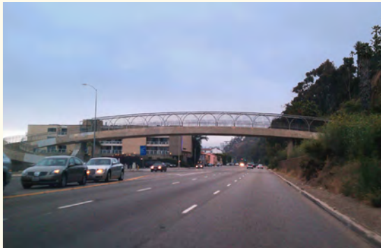
Pedestrian bridge and stairs at the California Incline
