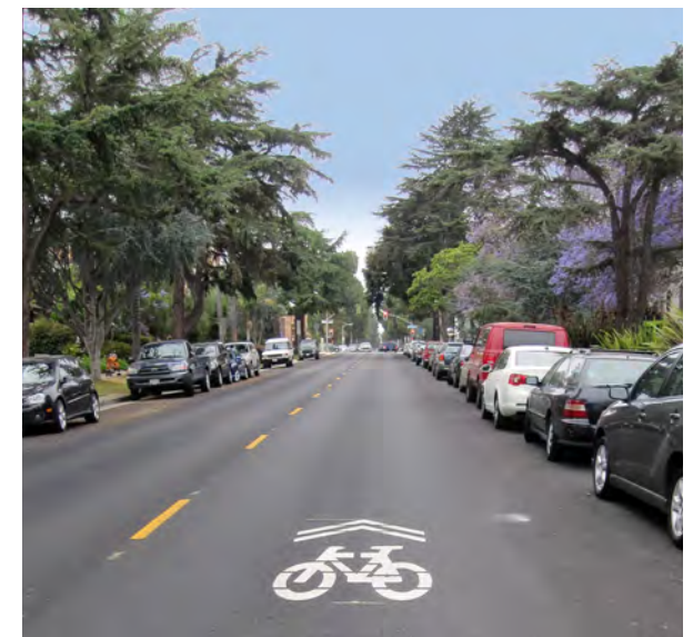
Shared lane markings installed on 14th Street in Santa Monica.
