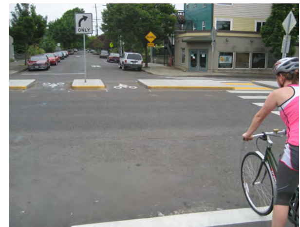
Traffic diversion (median barrier, shown above) is a common feature of neighborhood greenways. Source: Nelson\Nygaard
