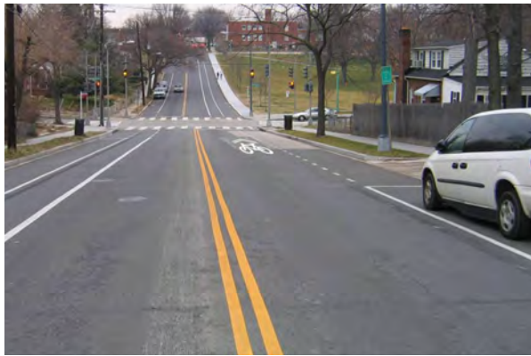
Climbing bike lanes: In Santa Monica, these would be enhanced with shared lane markings in the opposite direction. Source: Michael Ronkin
