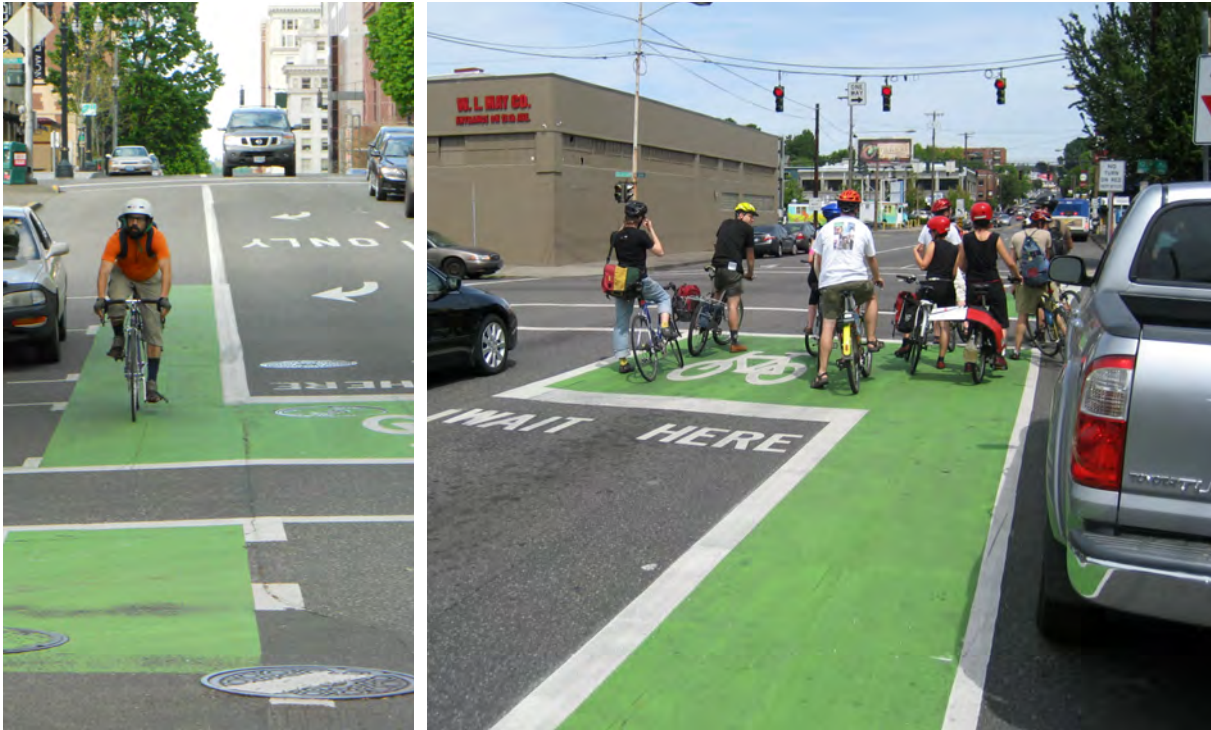
Bike boxes and colored bike lanes through intersections should be focused at high turn volume intersections. Source: Nelson\Nygaard (left) and Flickr user Cheryl & Rich, Creative Commons License 2.0 (right)
