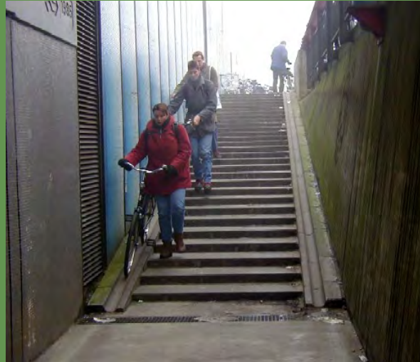
Stair troughs will greatly facilitate access to the beach at various bridge connections. Source: Nelson\Nygaard
