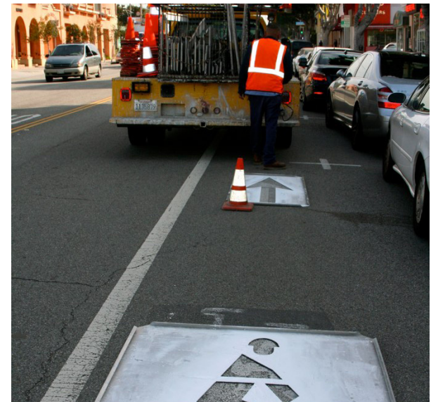
City crew installs bike symbols and arrows.
