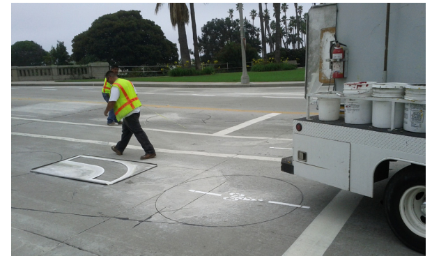
City crews install bicycle lane symbols and directional arrows.
