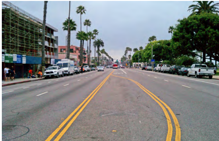
Existing Ocean Avenue between Broadway and Colorado
