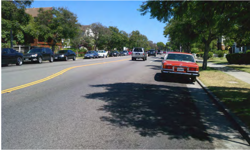
Existing 11th Street between Michigan and Pico
