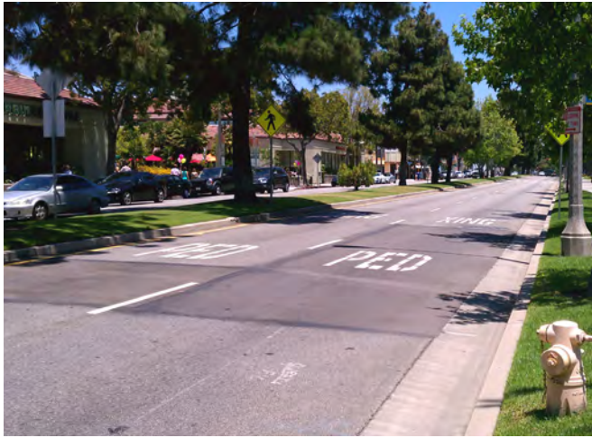
Ocean Park Boulevard's existing raised median between 29th and 30th Street
