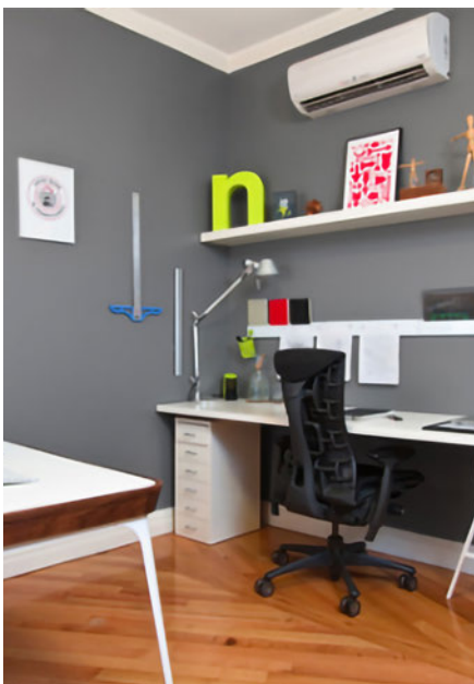
Ductless Heat Pump (Courtesy of Nick Keppol).
