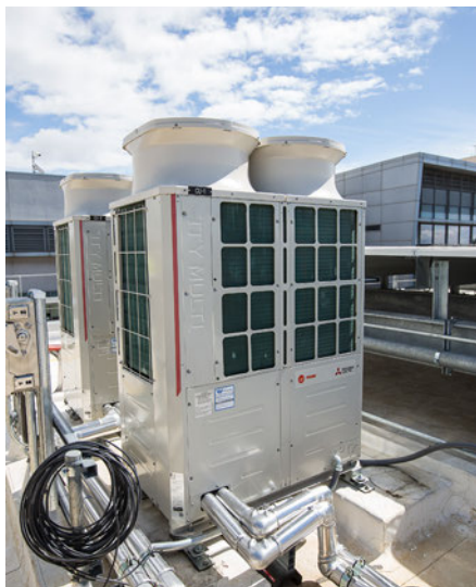
The outdoor unit for a commercial heat pump space conditioning system at the Santa Monica City Hall (Courtesy of City of Santa Monica).
