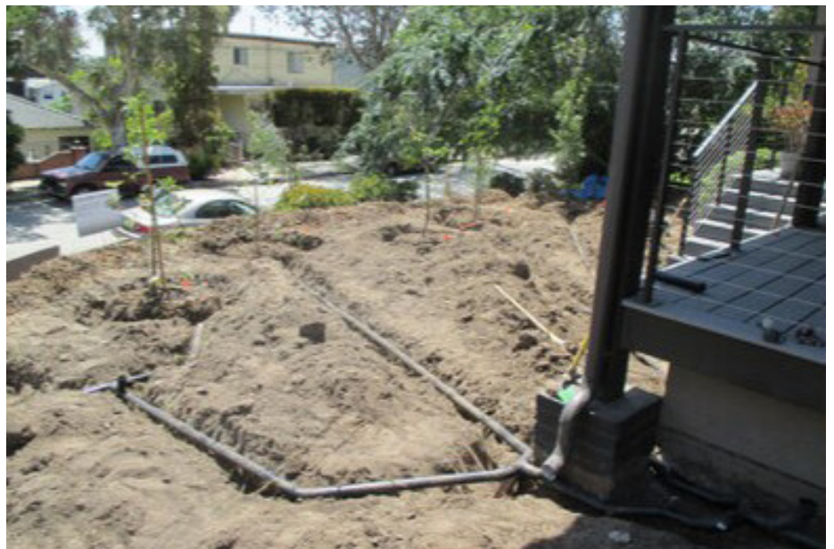
A greywater irrigation system is being installed in Los Angeles, CA. (Courtesy of Greywater Corps)
