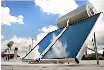
A solar hot water system uses less energy than electric resistance or a heat pump to heat water. (Courtesy of U.S. Department of Energy)
