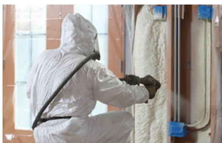
Spray foam insulation can increase comfort by minimizing heat transfer, reducing HVAC loads (Courtesy of Dan Tapia).
