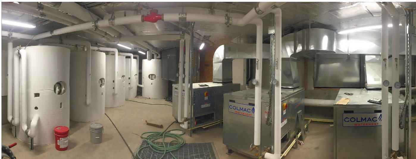
Central HPWH equipment with 2500 gallons storage located in a parking garage in the Batik Apartments, Seattle, WA (Courtesy of Ecotope).
