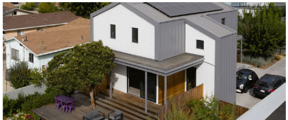
Perlita Passive House in Los Angeles, CA designed by Arcolution LLC. (Image courtesy of Lawrence Anderson)
