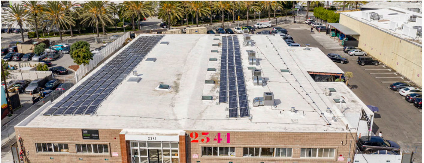
Rooftop solar with building-scale battery storage in Santa Monica (Courtesy RedCar)
