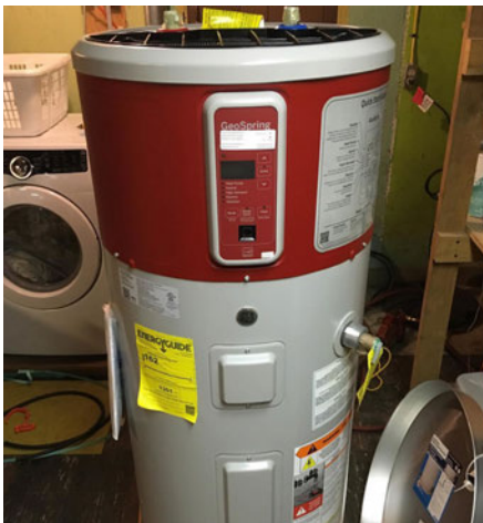
Individual heat pump water heater. The heat pump is located above the storage tank (Courtesy Jeff Robbins).
