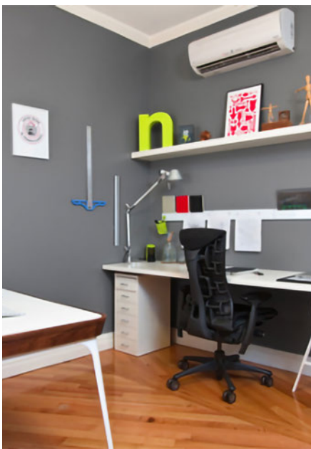
Ductless Heat Pump (Courtesy of Nick Keppol).
