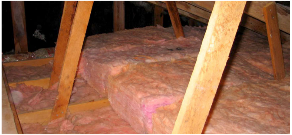
R-38 Attic Insulation. Photo by Ryan McFarland. www.zieak.com
