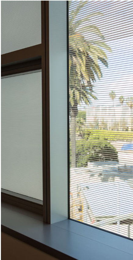
Blinds can be used to improve fenestration performance through reducing solar heat gain and glare. (Image courtesy of City of Santa Monica).
