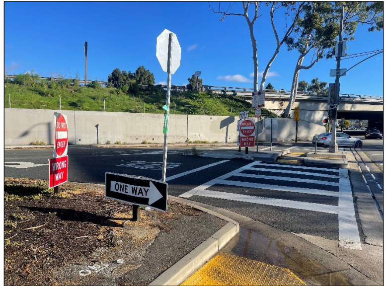
Figure 24 Pedestrian Crossing at I-10 Intersection
