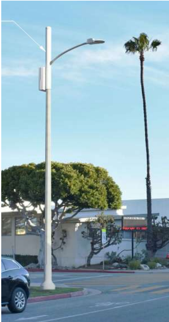
Figure 2: A photosimulation of a City-owned streetlight with a personal wireless service facility located at the northwest corner of 14 th St and California Ave. The backpack is mounted on the sidewalk-facing side of the streetlight and the antenna shroud extends down the length of the pole to cover all stainless steel banding. These design components meet the City's design standards. (Note: The color of the shrouds should be a darker gray to match the pole.) Other components, such as the WTR box, are installed below grade.
