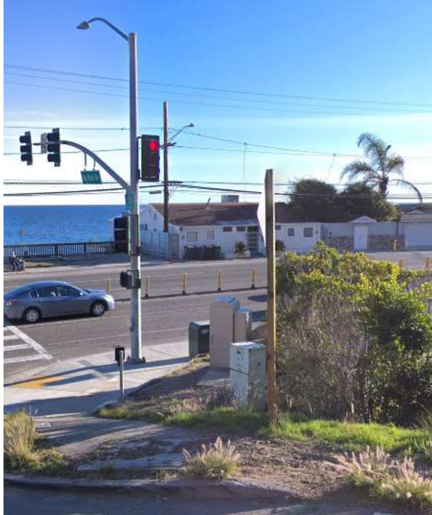
Figure 6: The traffic signal pole shown here supports side mounted traffic signals (at different elevations). A wireless facility is therefore permitted on this traffic signal pole.
