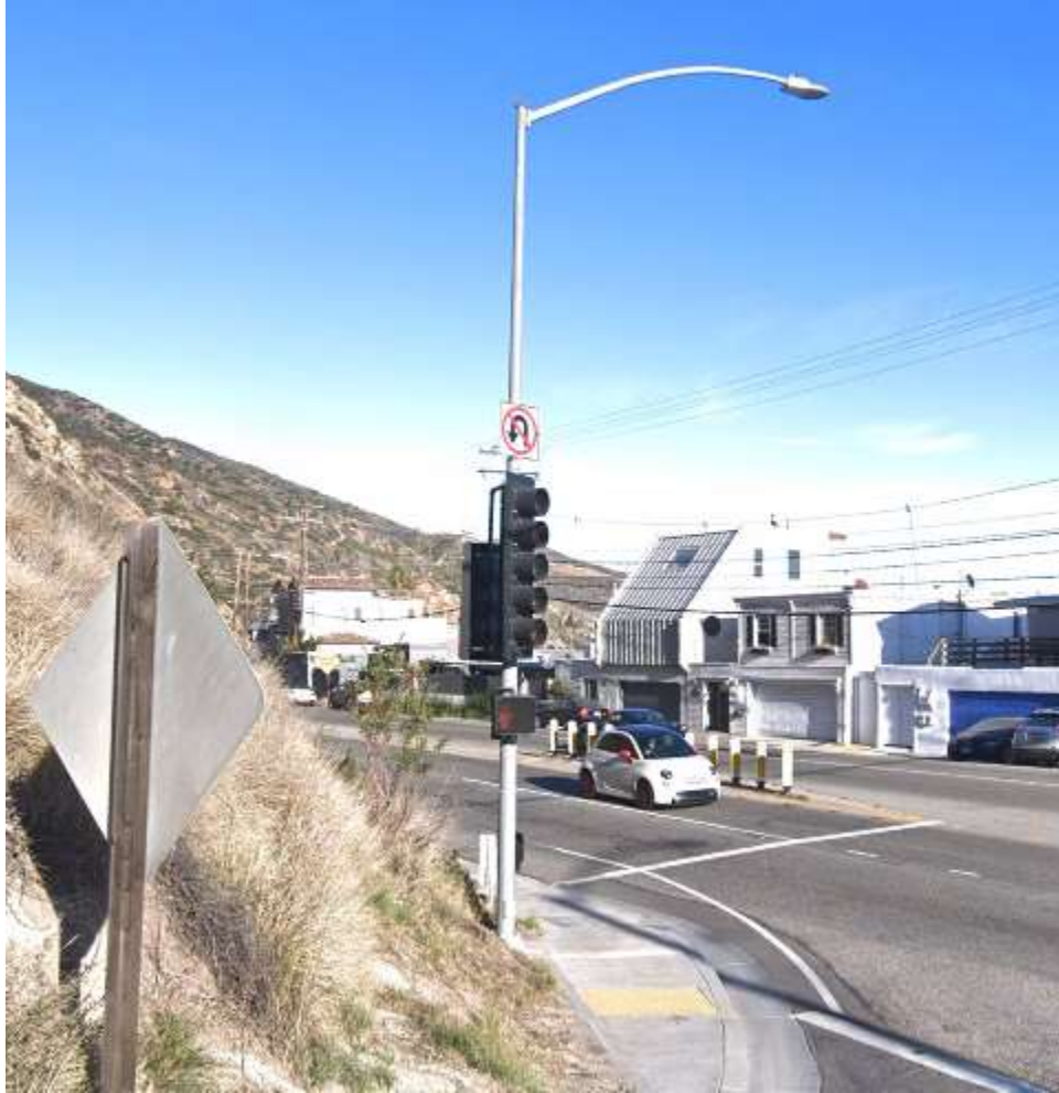
Figure 5: The traffic signal pole shown here supports side mounted traffic signals (below the No U Turn sign). A wireless facility is therefore permitted on this traffic signal pole.
