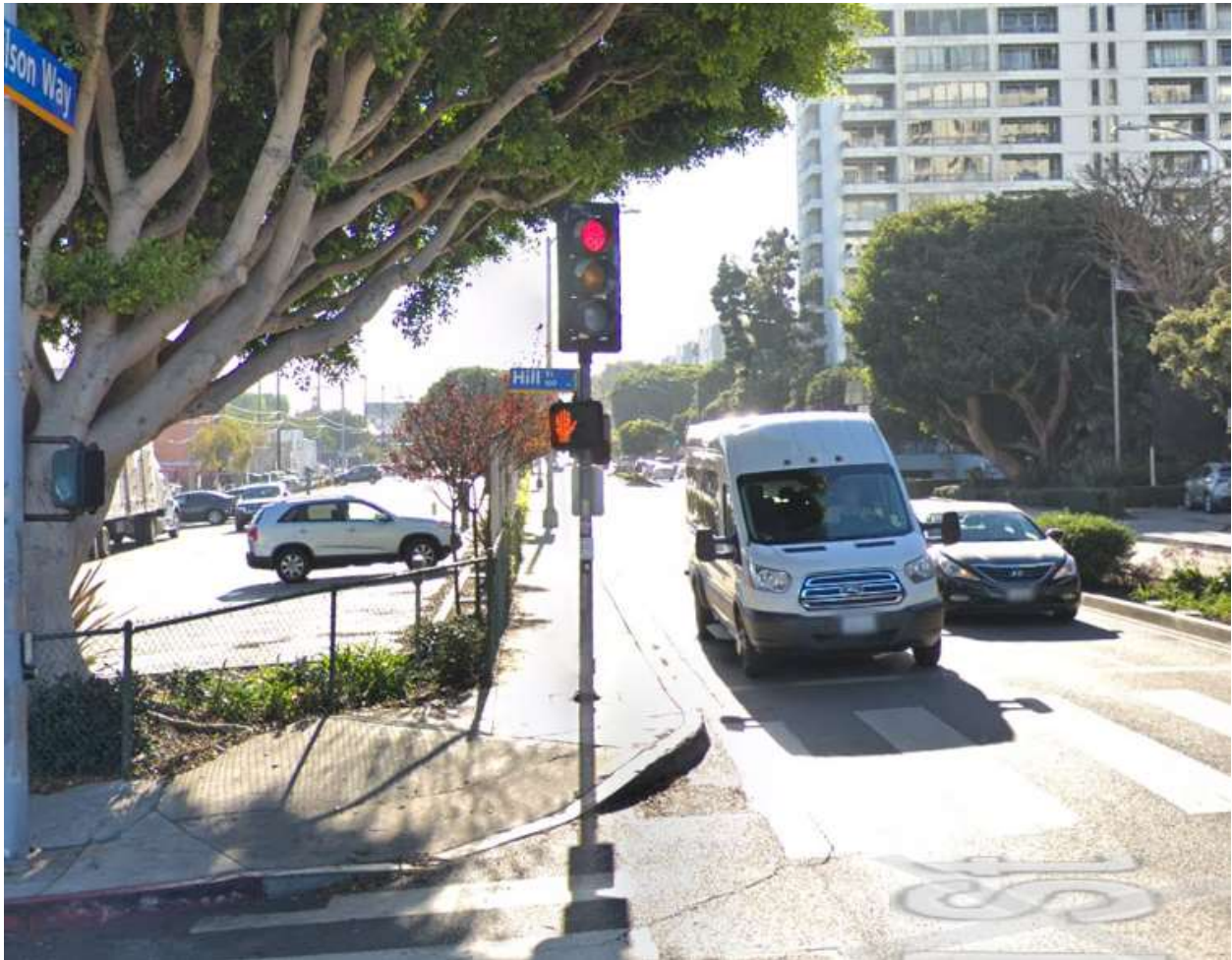
Figure 7: The traffic signal pole shown here supports a top mounted traffic signal. Installations of wireless facilities are permitted on traffic signals that support side mounted traffic signals. Therefore, installation of a wireless facility on this traffic signal is prohibited.
