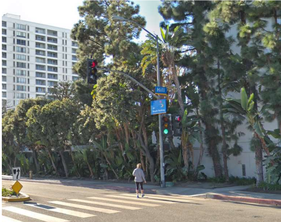
Figure 4: The traffic signal pole shown here supports side mounted traffic signals (below the street name sign). A wireless facility is therefore permitted on this traffic signal pole. Note that installation of a wireless facility on the mast arm of the traffic signal structure is prohibited.
