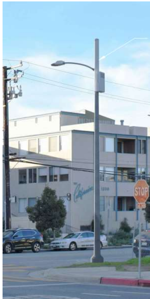
Figure 2: A photosimulation of a City-owned streetlight with a personal wireless service facility located at the northwest corner of 14 th St and California Ave. The backpack is mounted on the sidewalk-facing side of the streetlight and the antenna shroud extends down the length of the pole to cover all stainless steel banding. These design components meet the City's design standards. (Note: The color of the shrouds should be a darker gray to match the pole.) Other components, such as the WTR box, are installed below grade.
