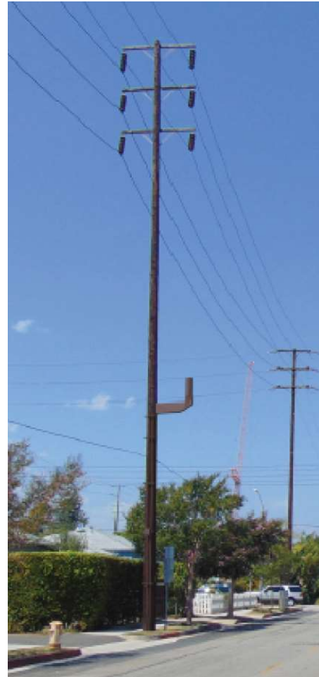
Figure 4: (Left) A photosimulation of a Joint Pole Committee utility pole with a personal wireless service facility located in front of the Appian Way frontage of 1711 Ocean Front Walk. The tubular design of the concealment shroud and antenna meets the City's design standards. Other components, such as the WTR box, are installed below grade. (Right) A photosimulation of a Joint Pole Committee utility pole with a personal wireless service facility located in front of 2320 20 th St. The integrated bracket arm meets the City's design standards. Other components, such as the WTR box, are installed below grade.
