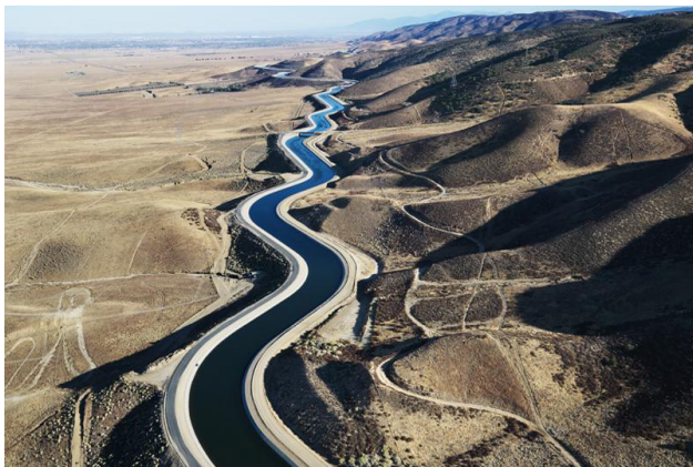
The California Aqueduct in the Central Valley.
