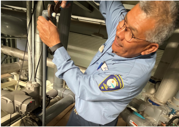
Operator performing preventative maintenance on plant equipment.
