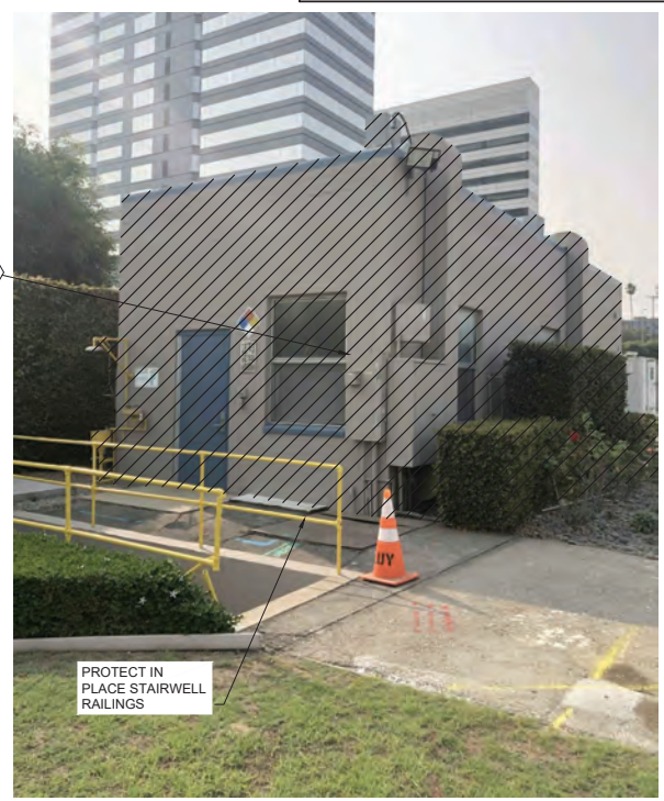
CHLORINATION BUILDING (LOOKING NORTHWEST)
