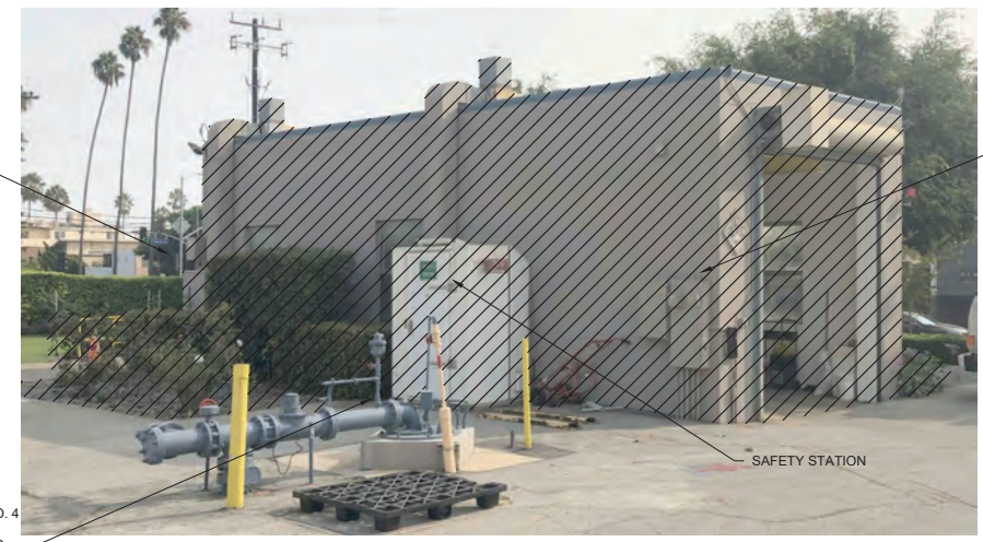
WELL NO. 4 AND CHLORINATION BUILDING (LOOKING SOUTHWEST)
