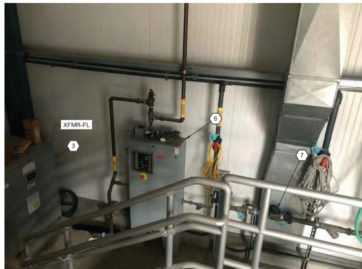
TEMPERED WATER HEATER AND BACKFLOW PREVENTER
