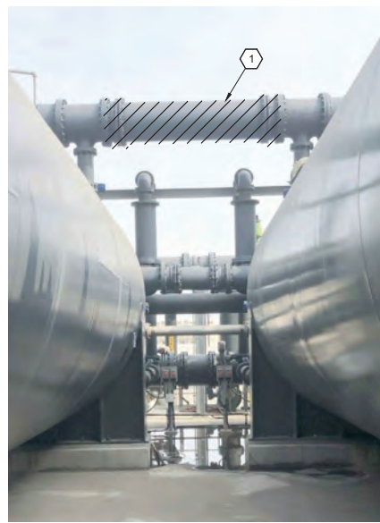
FLOW SEPARATION FOR PRESSURE FILTERS 5 AND 6
