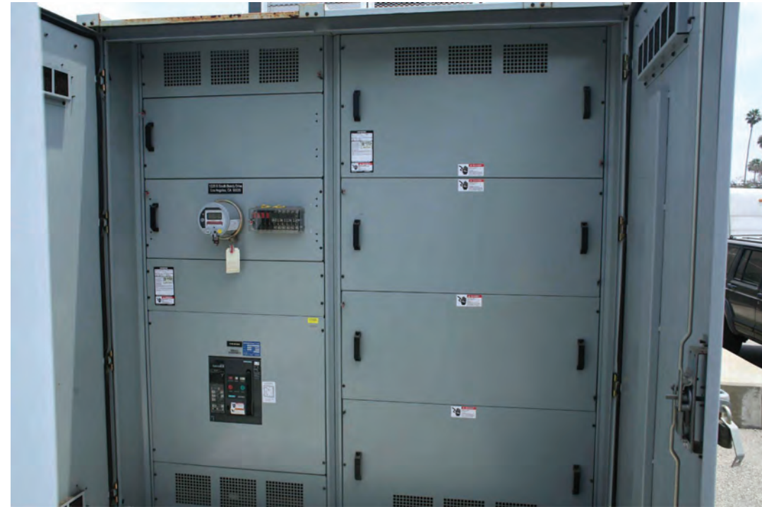
EXISTING SERVICE ENTRANCE SECTION- MS-RO
