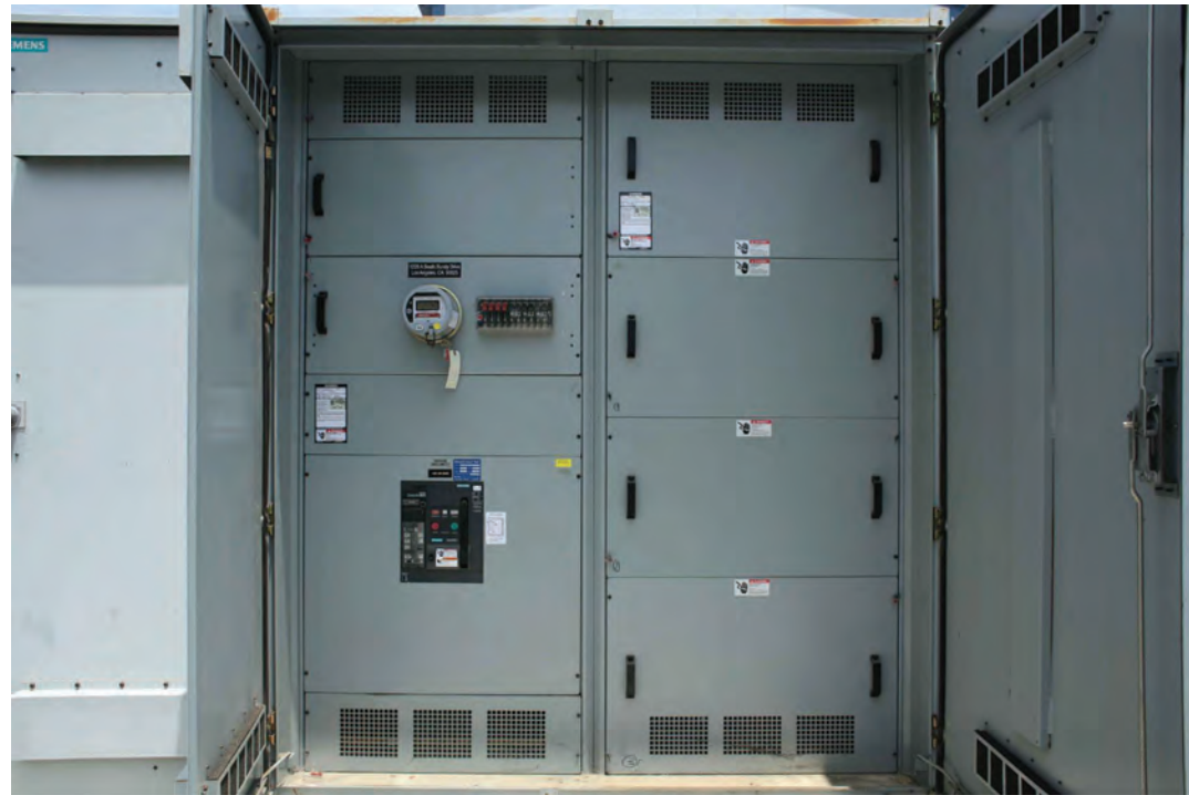
EXISTING SERVICE ENTRANCE SECTION- MS-A ①
