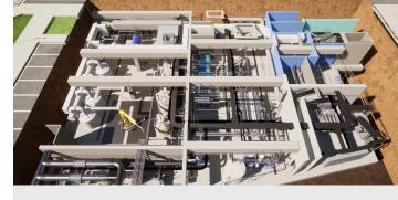
Located beneath the Civic Center parking lot, the SWIP AWTF will produce up to one million gallons per day of purified water for non-potable reuse (e.g., irrigation) and potable reuse to recharge our local groundwater aquifers.
