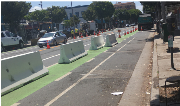
3. Main Street - parking is repurposed, concrete k-rail is added to serve as the parklet barrier
