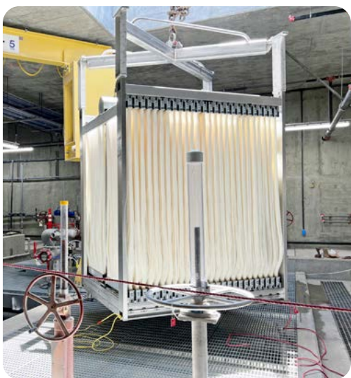
Ultrafiltration system being lifted from the surface at the SWIP
